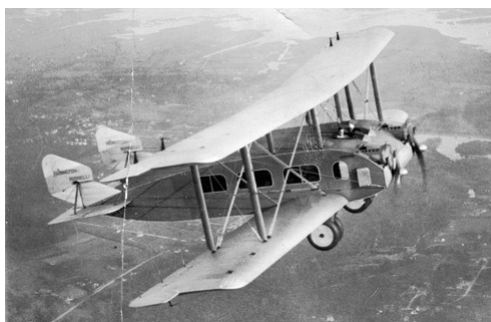
An early Burnelli lifting fuselage design. Compare with the futuristic designs on page 4
