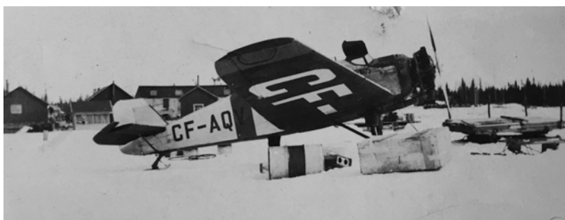
CF-AQV was a Junkers 33/34 owned by Canadian Airways. It crashed 5 miles SW of Gold Pines on September 1, 1939. It hit trees while low flying in poor weather. The remains are currently in the Deutsches Technikmuseum in Berlin. It is to be restored in Hungary and will go on display at the Technikmuseum when restoration is complete.
