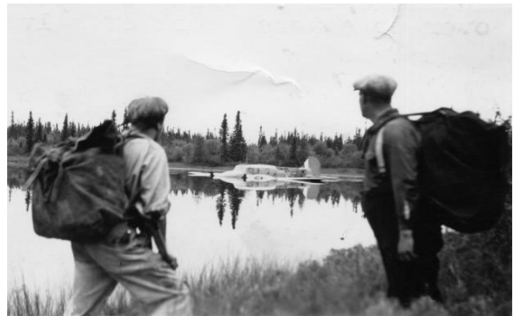
Packing equipment in to salvage the partially submerged Anson
