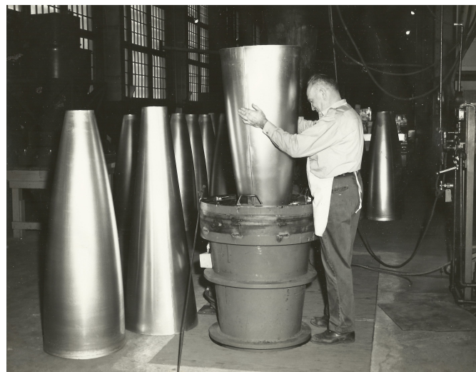
A bulge formed cone being removed from a mould
